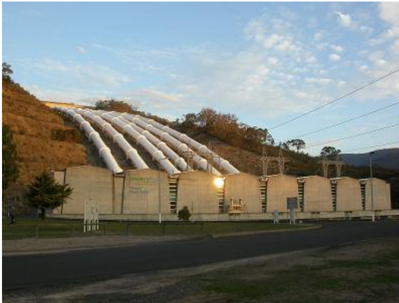
Tumut 3 1500 MW pumped hydro storage system in the Snowy Mountains © A Blakers
