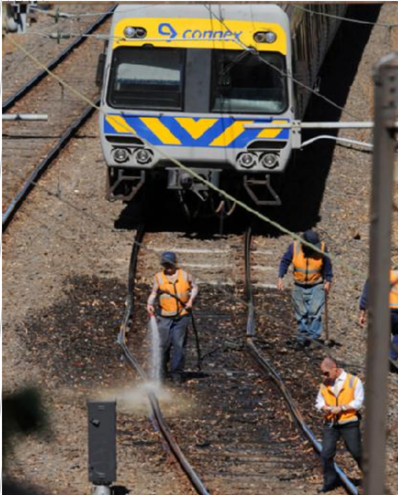
Melbourne Rail Buckling - The Age, Jan 29, 2009
